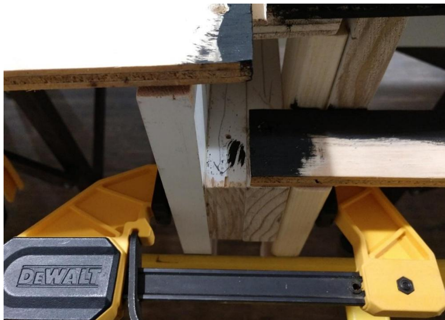
Fascia 4 – Mounting fascia support (white vertical 1x3) to 1x3 cross braces
