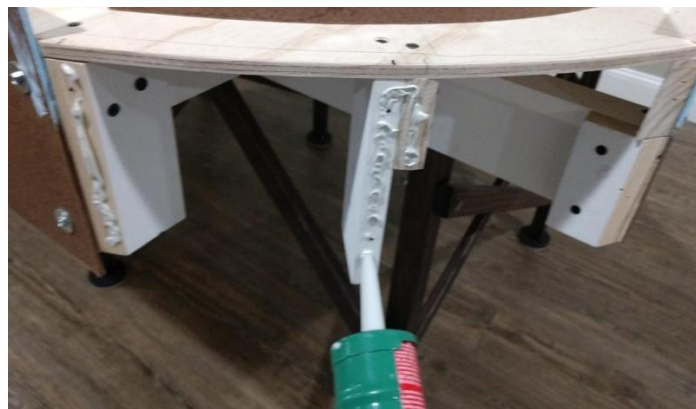
Fascia 18 – Applying Liquid Nails construction adhesive to fascia supports
