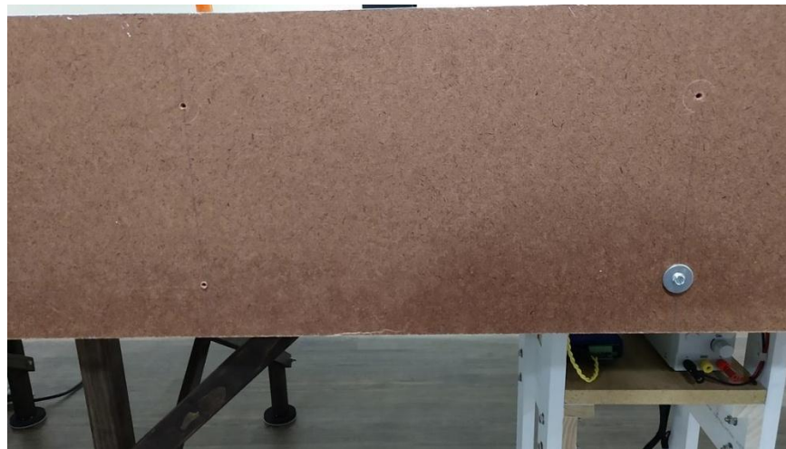
Fascia 21 – Removing screws and washers from fascia
