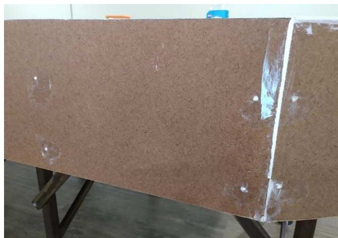
Fascia 22 – Using spackling baste to fill in screw holes and gaps in fascia
