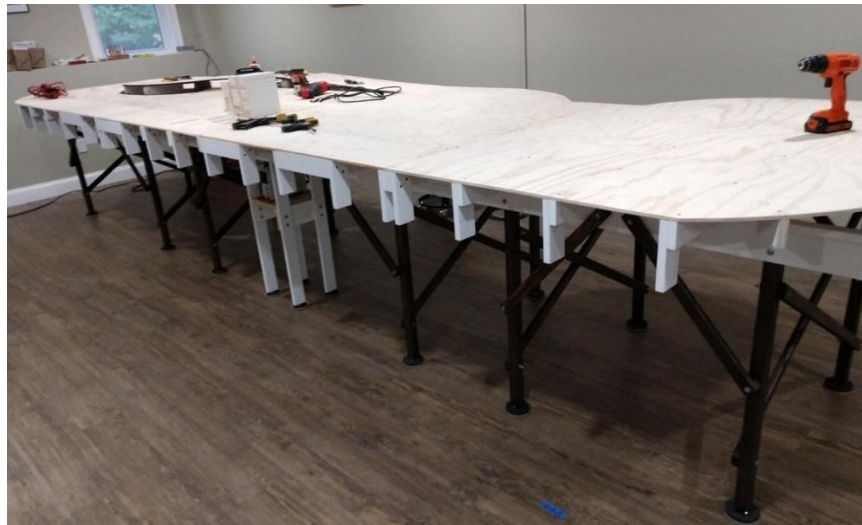
Fascia 2 – Fascia support pieces extending down from 1x3 cross braces
