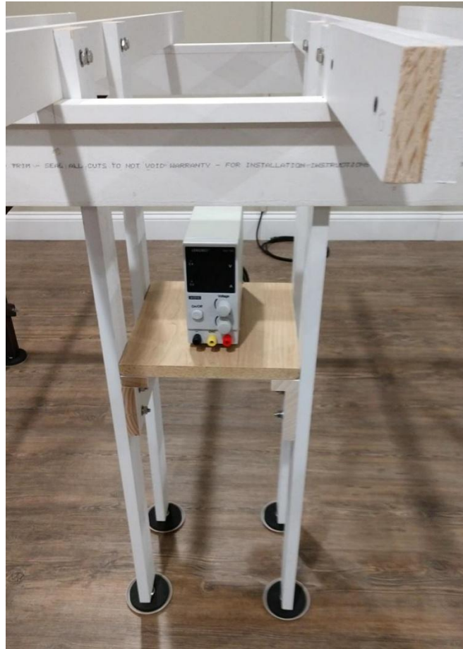
Shelf 1 – Front view of power supply shelf
