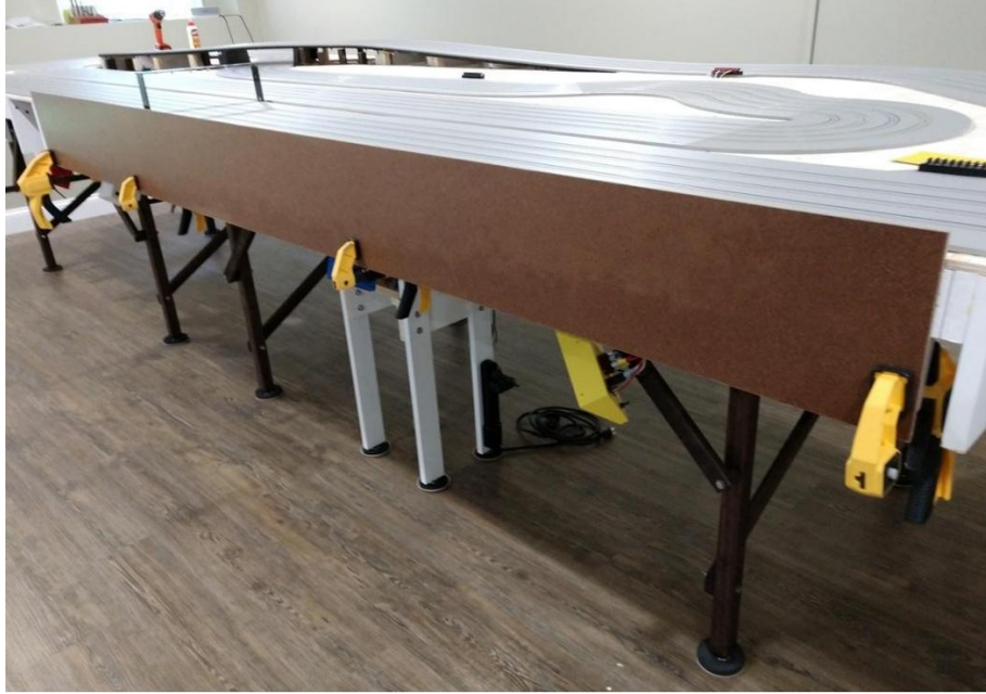
Fascia 7 – Initial fitting of fascia section using clamps
