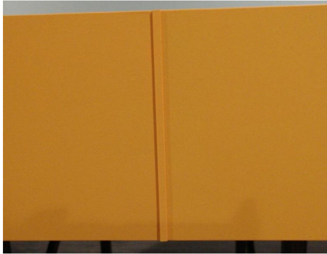
Fascia 32 – Plastic “T” inserted into fascia gap
