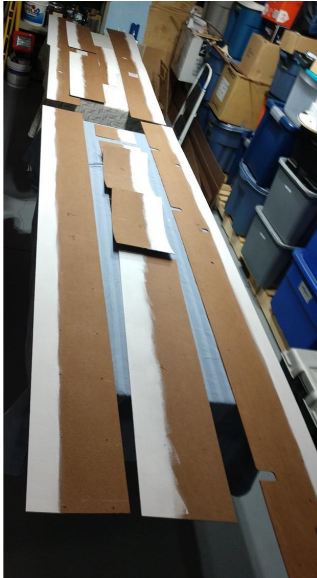
Fascia 13 – Inside top portions of fascia sections painted with primer
