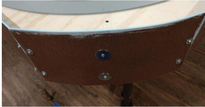
Fascia 19 – Fascia section mounted using screws and washers
