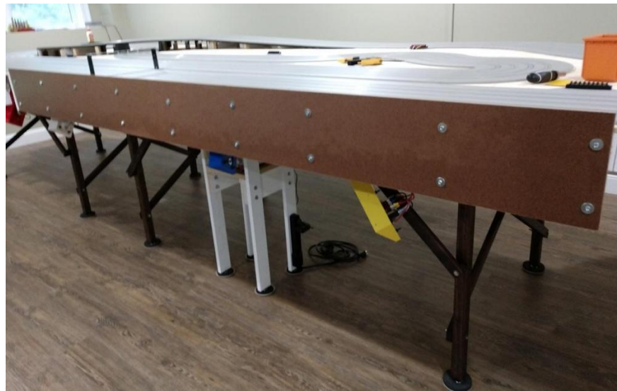
Fascia 8 – Fascia section temporarily mounted using screws and washers
