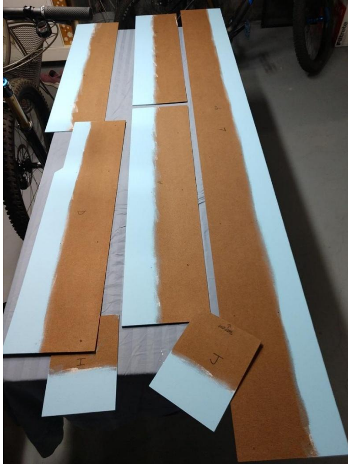
Fascia 14 – Fascia sections painted and ready for final installation
