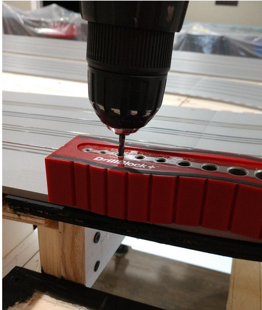
Secure 2 – Using DrillBlock jig to drill track mounting hole
