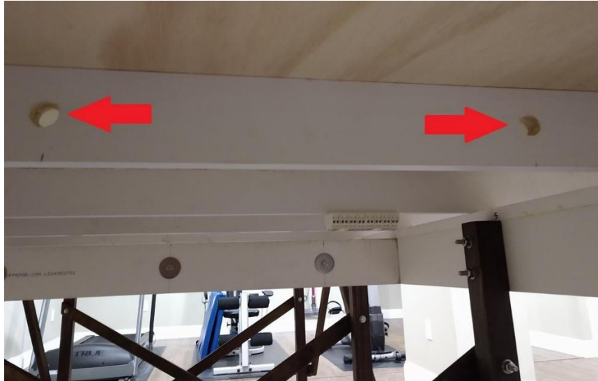
Wiring 4 – Wiring feed thru holes underneath benchwork
