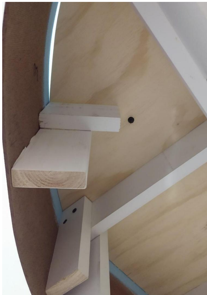
Fascia 20 – View of Fascia attached to benchwork from underneath
